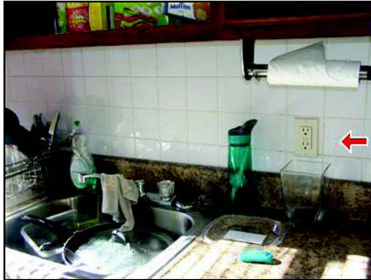
8.5 Picture 1 GFCI outlets in 2nd floor kitchen.
