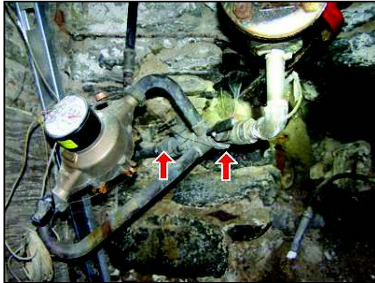
7.3 Picture 1 Potable water shut off valves
