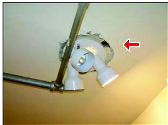
4.0 Picture 5 Fifth floor kitchen light not installed properly
