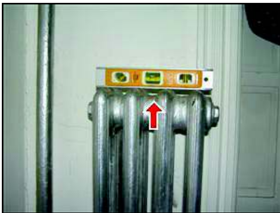
9.4 Picture 2 Radiator in 4th floor front room pitched wrong way
