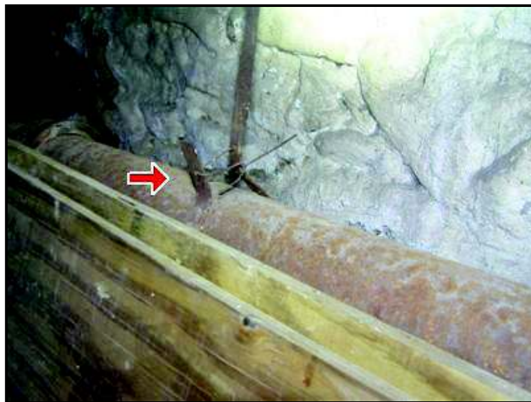
7.0 Picture 2 Hanger bracket not secured properly
