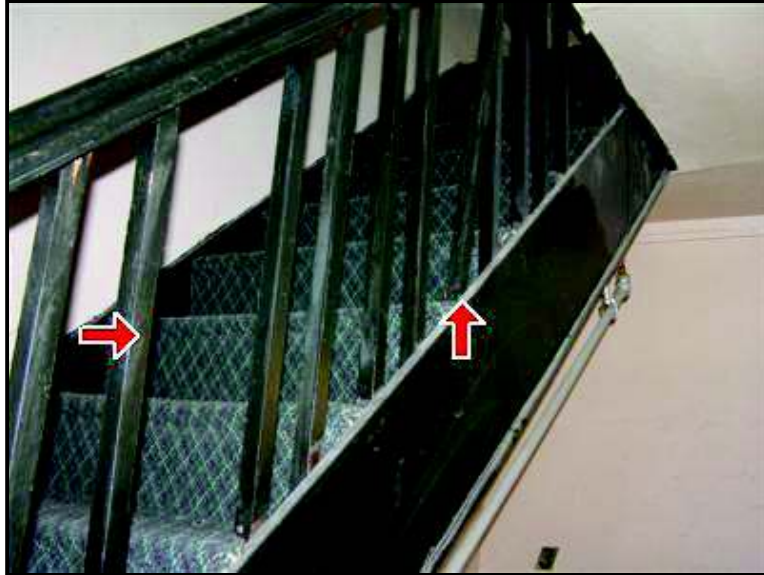
4.3 Picture 1 Missing & loose baluster
