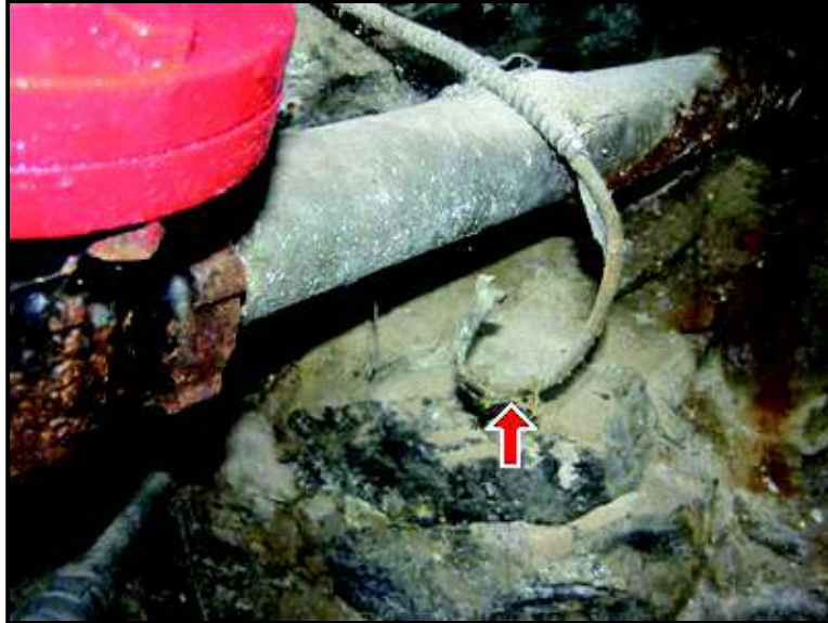
8.1 Picture 1 Ground not secured to water main
