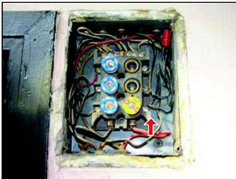
8.1 Picture 2 5th floor panel, fuse doubled lugged
