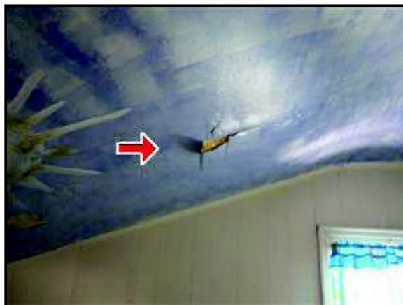
4.0 Picture 2 Middle bedroom plaster cracked and peeling
