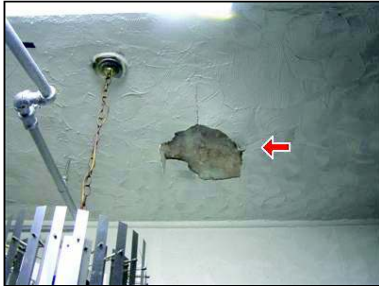
4.0 Picture 3 Front bedroom plaster cracked and peeling
