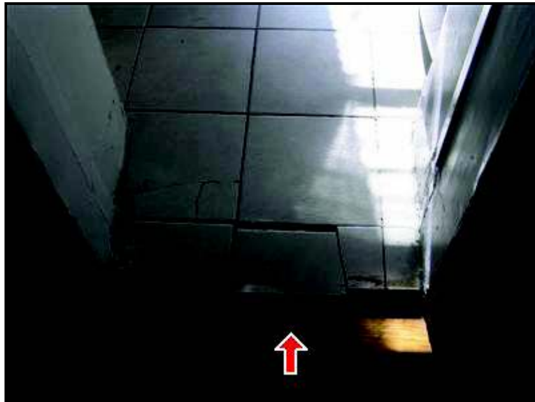
3.2.B Picture 1 Ceramic tile cracked.
