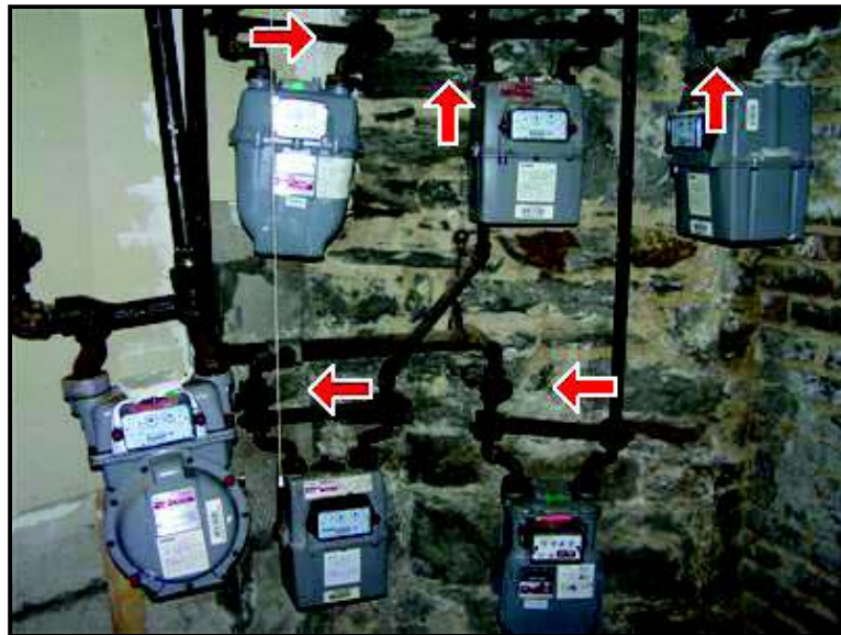
7.5 Picture 2 Apartment gas valves at meters
