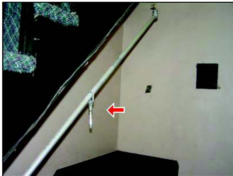
7.1 Picture 2 Support eye pulled out o
