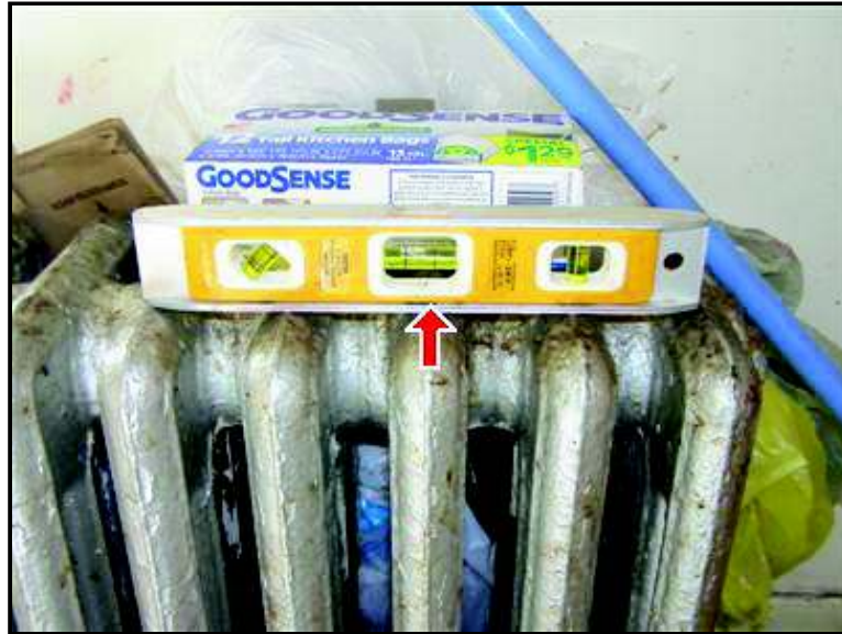
9.4 Picture 1 Radiator, 5th floor kitchen pitched wrong way
