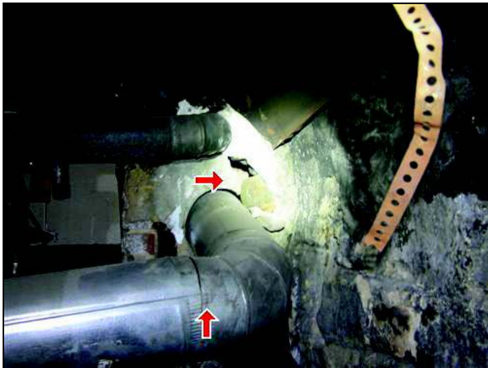
9.5 Picture 1 Open joint and chimney repair
