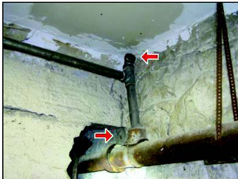
7.0 Picture 2 Hanger bracket not secured properly
