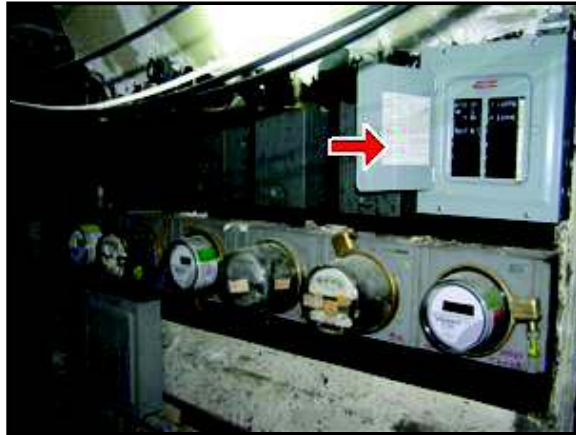
8.6 Picture 1 Main panel and meters
