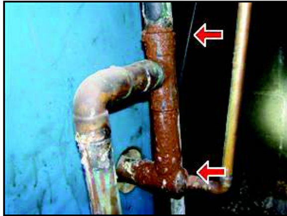
9.3 Picture 1 Leaking condensate return
