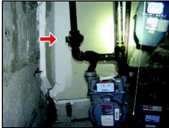
7.5 Picture 1 Hole house gas valve
