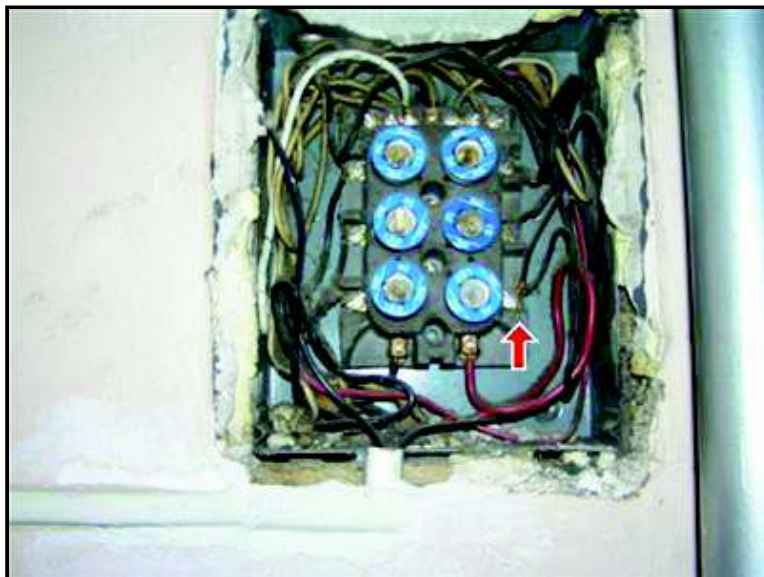
8.1 Picture 3 4th floor panel, fuse double lugged
