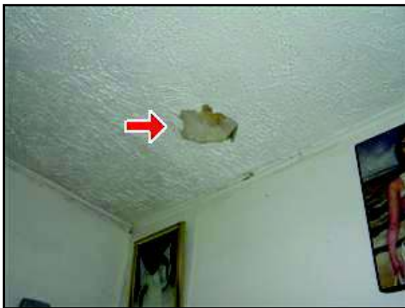
4.0 Picture 4 5th floor dining room plaster cracked and peeling
