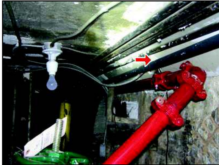
7.1 Picture 1 1" water pipe not supported
