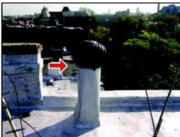
1.3 Picture 1 Passive turbine vent for bathrooms
