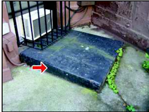
6.6 Picture 1 Basement vent cvered
