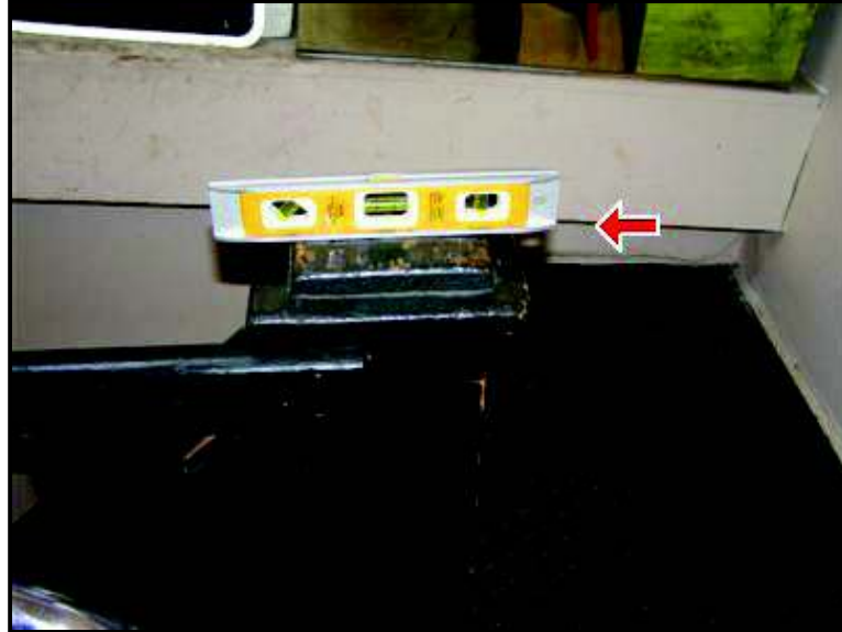
4.3 Picture 3 Fifth floor landing and railing pitched
