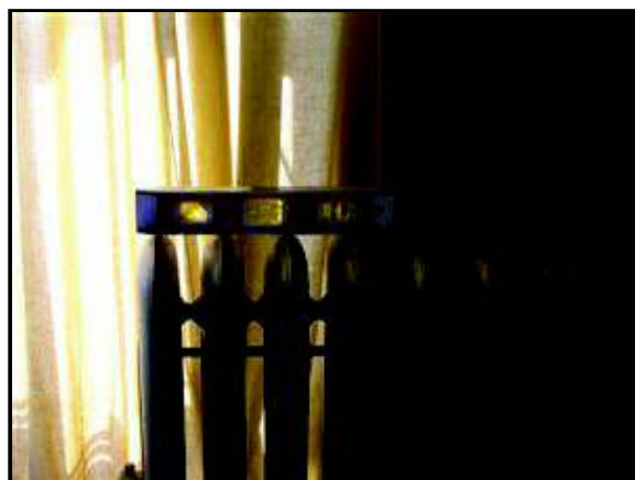
9.4 Picture 4 Radiator in 3rd floor bedroom pitched wrong way
