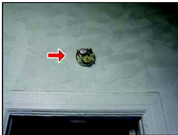
8.7 Picture 1 Battery missing 3rd floor apt.
