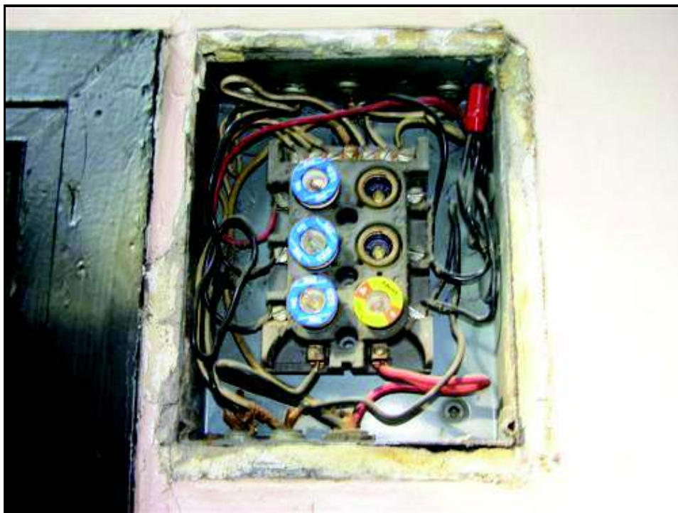
8.6 Picture 2 5th floor panel
