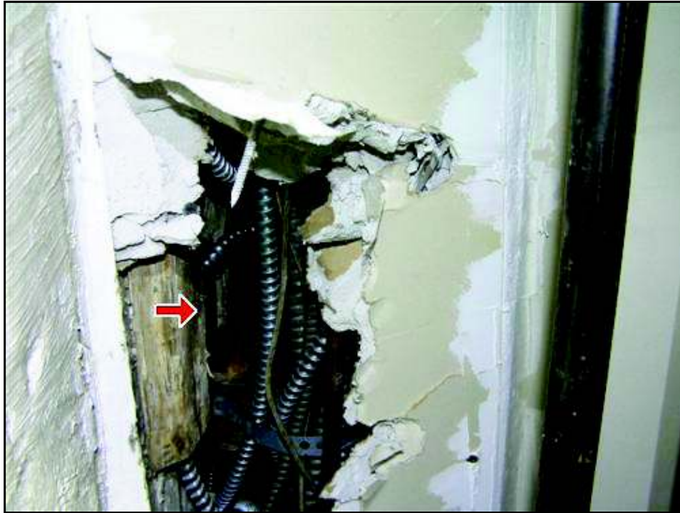
6.3 Picture 1 3" x 8" floor joists
